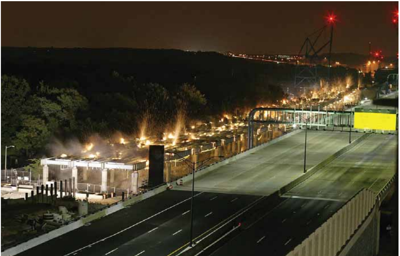
Photo courtesy of Trevor Wrayton, Virginia Department of Transportation.
