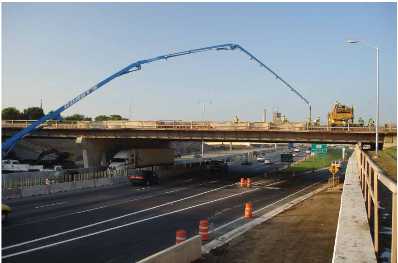
Construction of the Marquette Interchange underway in Milwaukee, WI.
