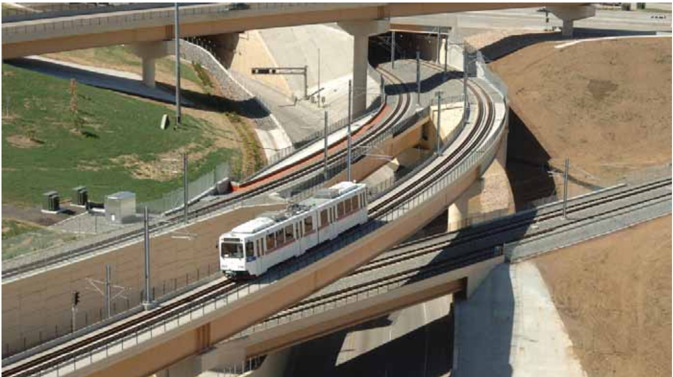
Southeast Light Rail Interchange opened as part of T-REX in Denver.
